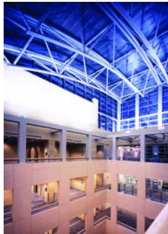
The spectacular five-story central atrium is a dramatic intersection of the three major building sections.
