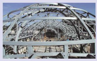
deel splices consisted of 32, 5/8"-dia. Hollo-Bolts at each splice. "Hole size and alignment was a must for the bolts to work," Brewsaugh said. "The erection of this frame was a challenge in the fact that the connections had to be pulled tight and clamped before inserting and torquing the bolts."
