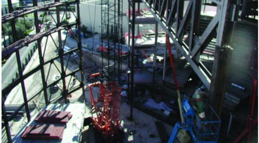
The crane was placed in a hole 25' below ground level and below the area of steel delivery. Trusses were sent to the jobsite in three pieces and assembled in the "hole" while the raising gang was erecting steel in the rest of the building.
