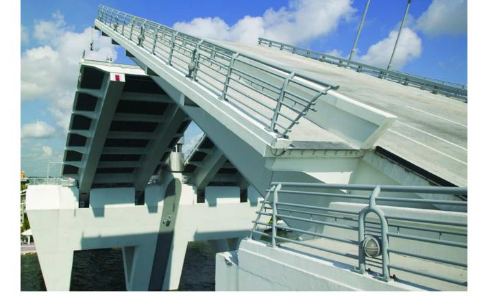
is curved to tuck below the cantilevered machinery floor with the bridge in the open position. Curved internal diaphragms transfer loads to the transverse diaphragms, which carry weight to the main girders. The box also eliminates the need for substantial falsework over the water, since its design supports the weight of the steel ballast and concrete.
