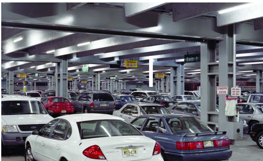
Below: The painted structural steel frame provides large spans and vertical clearances necessary to facilitate easy navigation.
