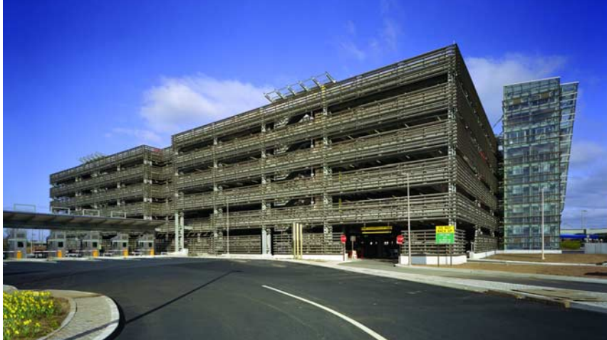
Above: The garage features a steel superstructure with an architectural metal screen-wall system enclosing the exterior façade.
