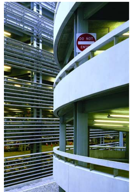
The double-helix ramp was constructed with high-strength cast-in-place concrete on an exposed steel frame structure.
