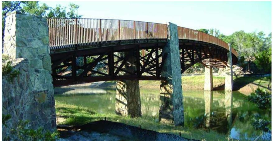
In designing the Spanish Oaks Golf Course Bridge at Hole #18, the landscape architect envisioned a structural steel pedestrian/golf cart bridge spanning over a man-made reflecting pond. The end result was a variable-depth arched-steel truss spanning to limestone-clad bents and abutments.
