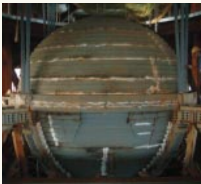
Above: The main tuned mass damper is composed of 730 tons of stacked steel plates.
