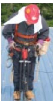
The Hilti ST 1800/SDT 25 Stand-Up System fastens deck-side laps and deck to thin bar-joist applications. It includes the ST 1800 Adjustable Torque Screwdriver, SDT 25 Stand Up Tool, and collated screws matched to application needs. A magazine allows the user to fasten 50 screws before reloading for time saving. With its two-handle design and low vibration grip, it provides operator comfort. Hilti offers customer service, including submittal packages and job-site training.
