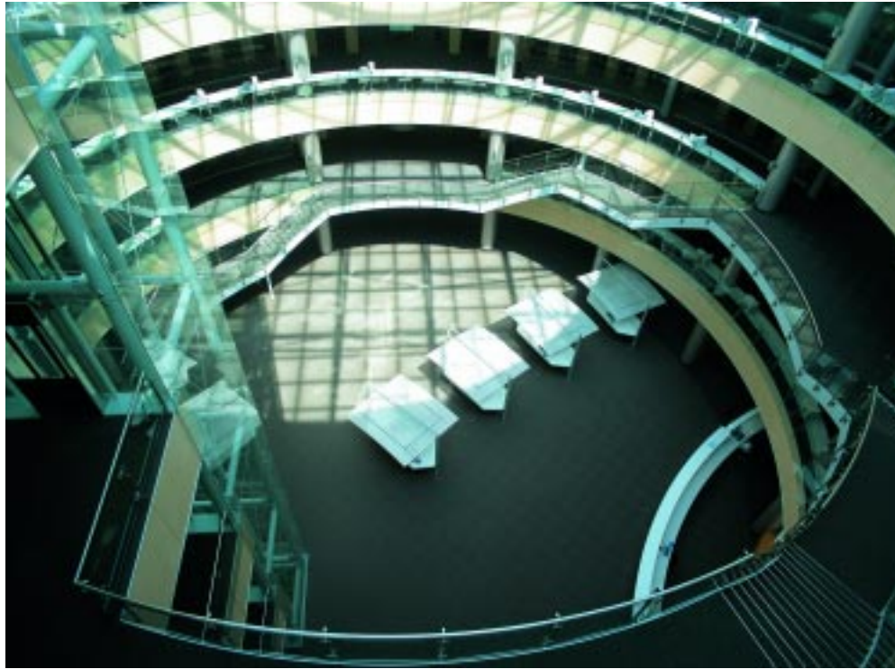
The glass-roofed central atrium is five stories high. Stainless steel and glass are combined to create a monumental stair connecting all levels of the digital library.
