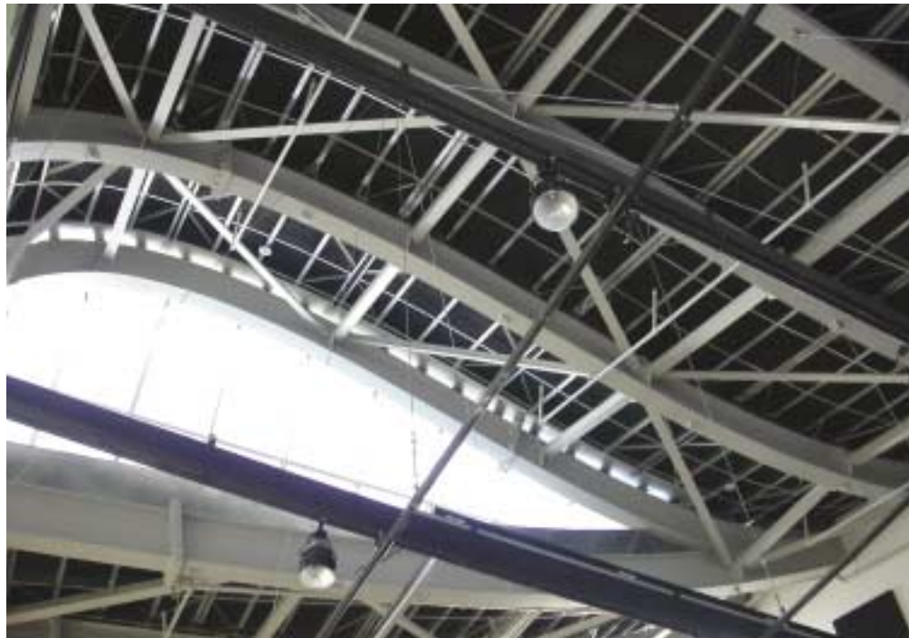
Below: Interior view of the "eyelid" in the Drama Room.
