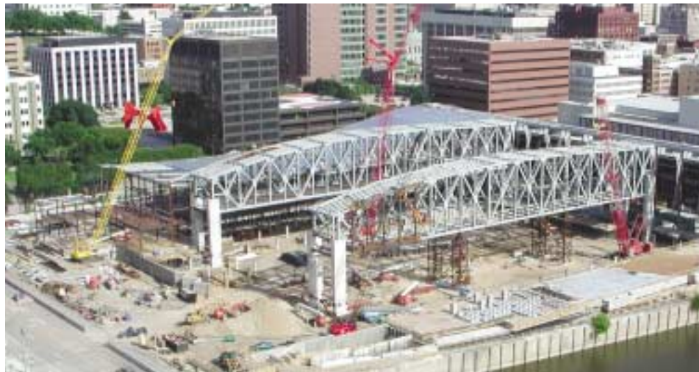
Above: Shoring towers, located at the third points along the span of each box truss, were used for the erection of the box trusses.
