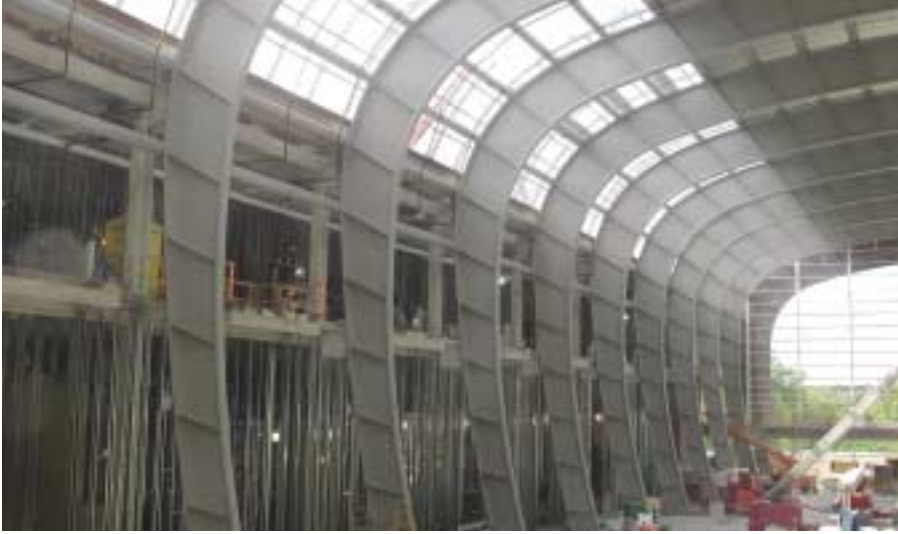
Interior view of the Grand Gallery during construction.
