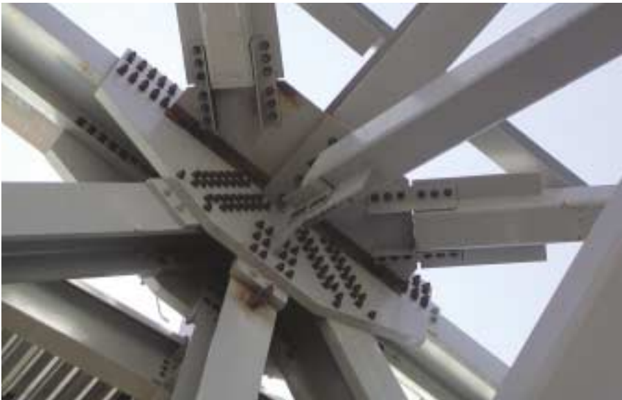
A box-truss top-chord connection
