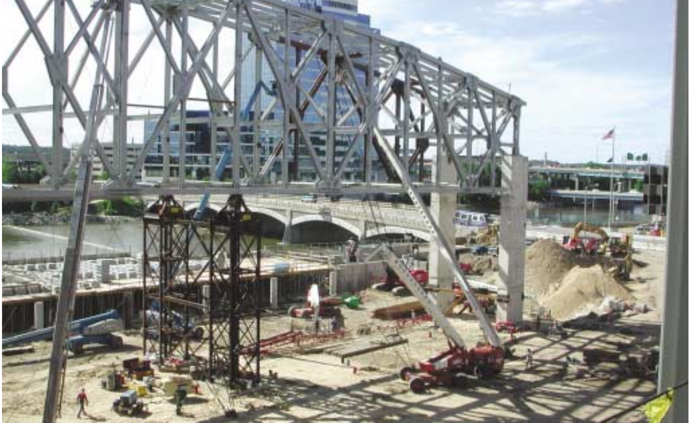
Above: Shoring towers, located at the third points along the span of each box truss, were used for the erection of the box trusses.
