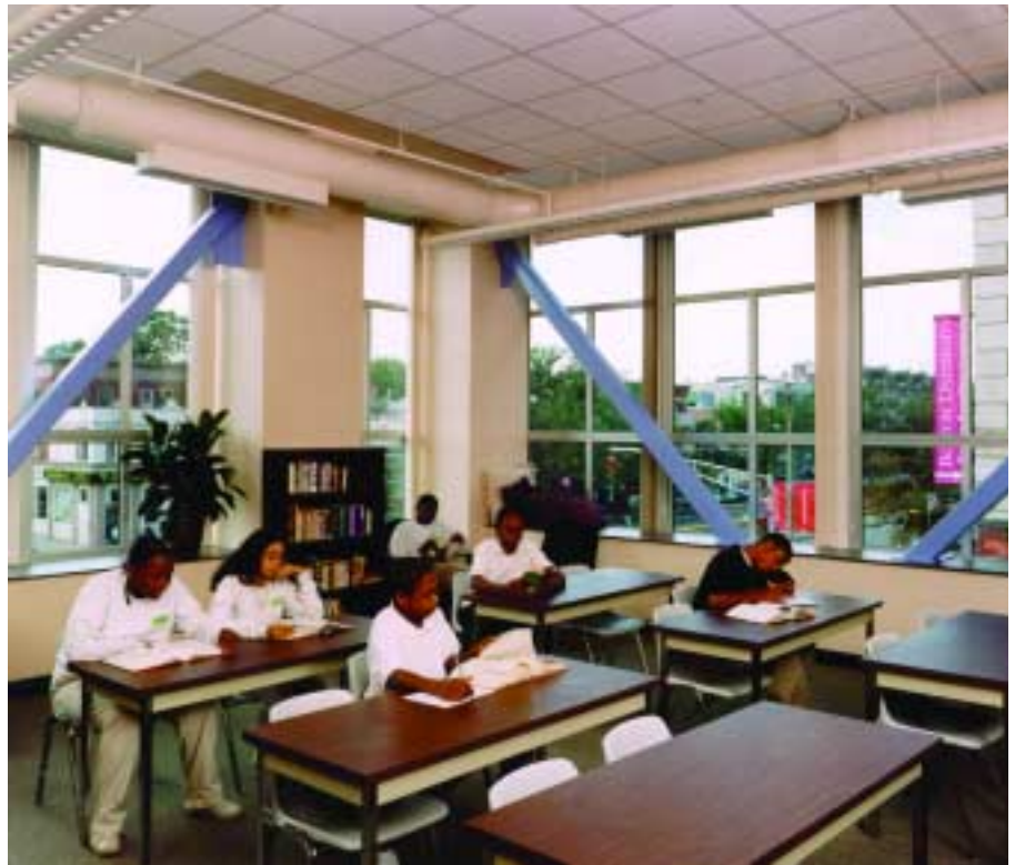
Above: New lateral bracing was installed along exterior column lines rather than interior column lines to maximize the flexibility of interior spaces.
