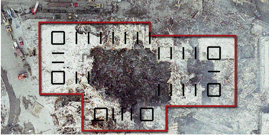
Collapse of World Trade Center 6, induced by falling debris from the North Tower. Note that the dark lines indicate approximate locations of one-bay steel moment frames around building perimeter.
