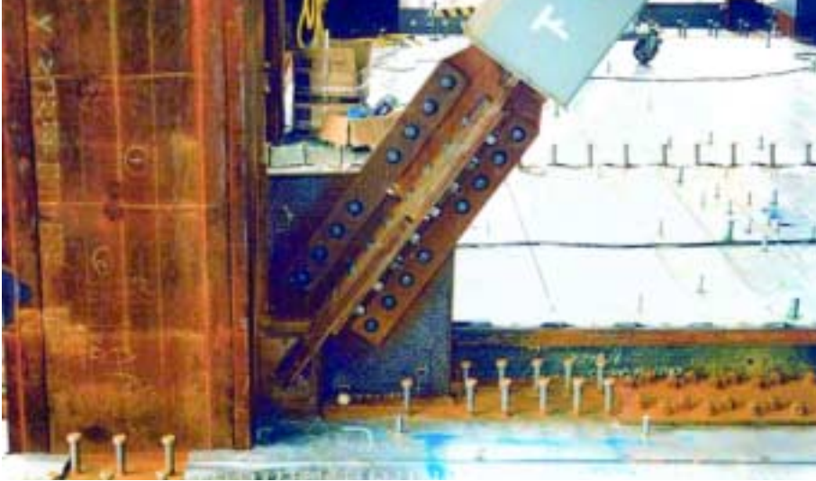
Buckling-restrained brace gusset connection.
