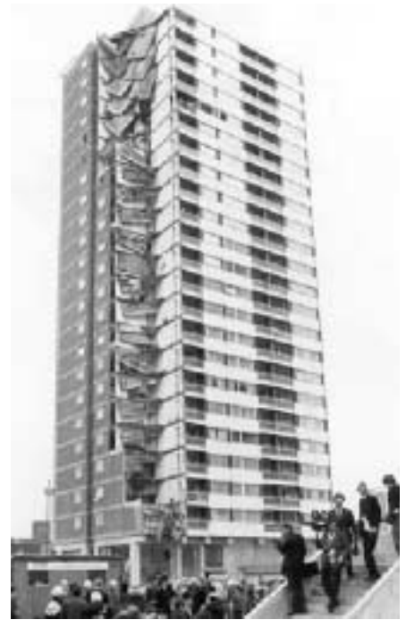
Ronan Point building after the May 1968 collapse.
