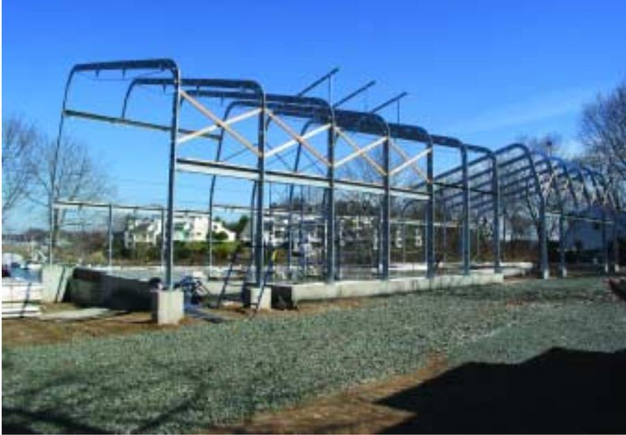
board, computer-milled to specification and delivered to site. Typically they are used either as an insulating skin over self-supporting timber frame, or at smaller scales as structural envelopes. When coupled with a steel frame and allowed to work structurally, large volumes can be contained efficiently. For this project, curved SIPs were developed for the first time, and were used for transitions at peaks and eaves. SIP Clips™ were developed to translate loads be-
