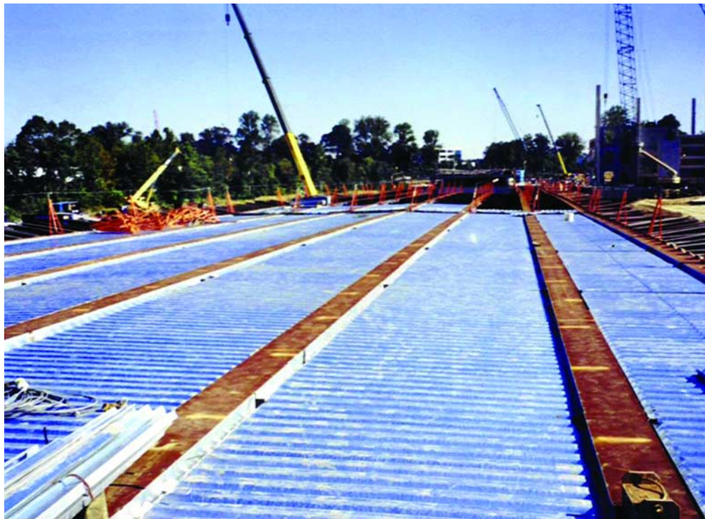
Below: SIP metal forms were used in the construction of the deck.
