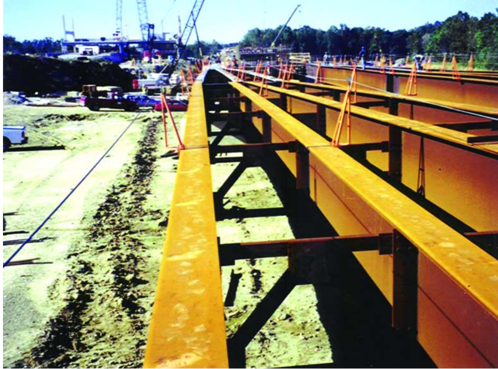
Above: ASTM A709 Grade 50W steel was used for all superstructure components.
