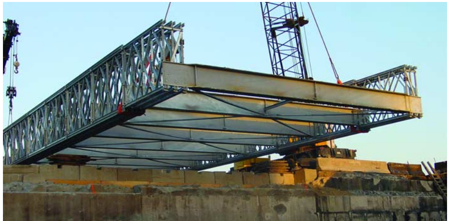
A temporary highway bridge supplied by Acrow Corporation is lifted into place to restore traffic flow on I-95 in Bridgeport, CT.
