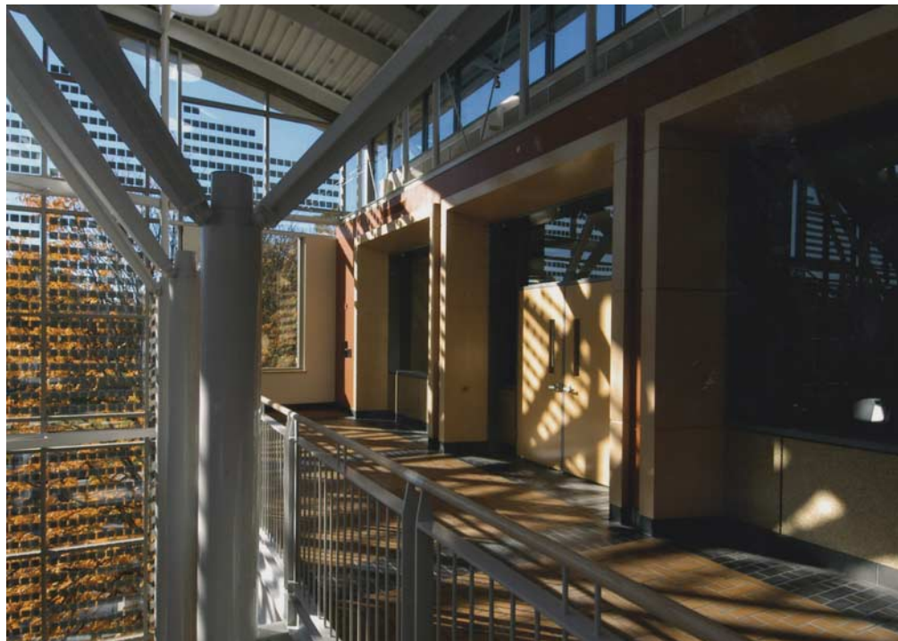
Above, center, and below: The exposed curved roof structure of the central atrium is supported by "tree" columns composed of round HSS "trunks" with "branches" of tapered \frac{3}{8} " plates welded into a cruciform cross-section.
