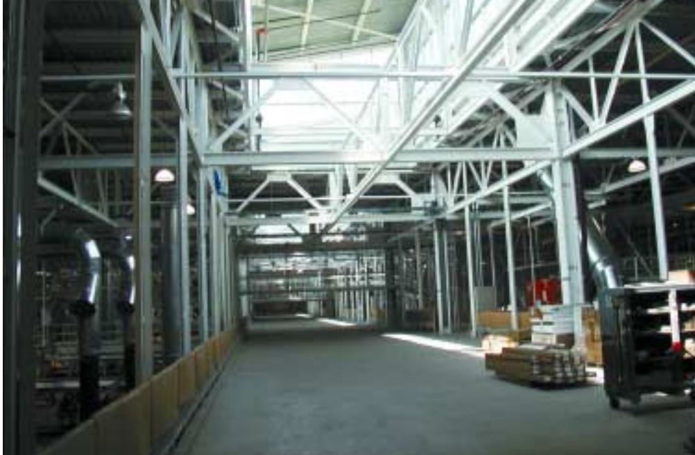
Light monitors placed over the employee mezzanine areas and exposed steel framing painted white help promote an invigorating work environment.
