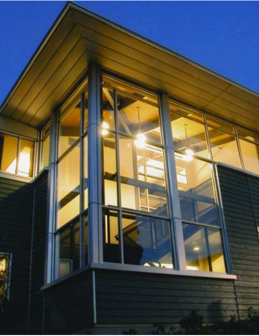
Smaller windows on the building's south side bring in daylight but block direct penetration of sunlight. Larger windows are placed on the northern exposure to capture cooler air for natural ventilation. Photo © Rick Keating Photography
