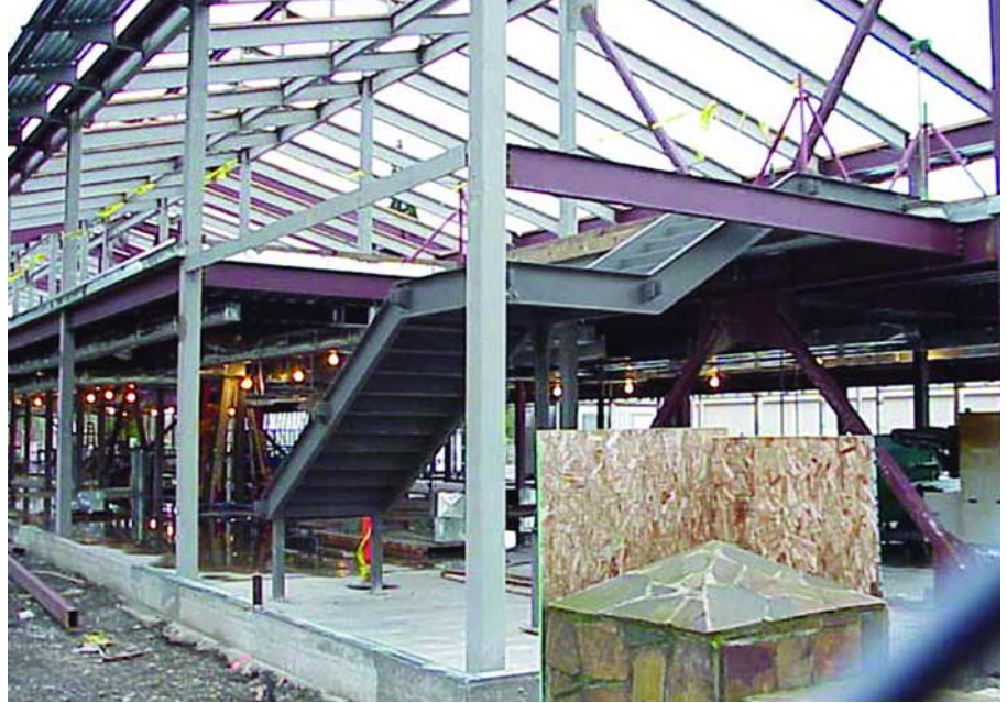
The ground floor is slab-on-grade construction.
