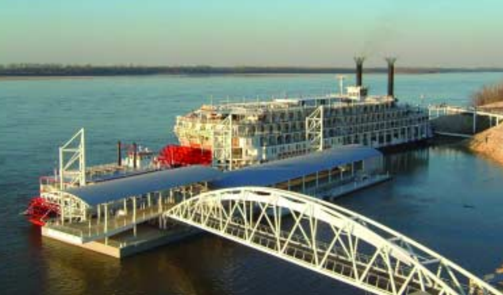
The floating steel dock rises and falls with the river level. A 200'-long hinged HSS truss gangway connects the dock to dry land. (Photo courtesy TetraTech, Inc.)
