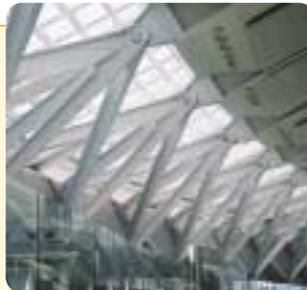
CAFCO SprayFilm – WB 4 Intumescent Fire Protection Coating is the first water-based thin-film intumescent fire-protection coating for structural steel approved by Underwriters Laboratories, Inc. (UL). SprayFilm – WB 4 does not require any reinforcement (i.e. glass fiber mesh and/or adhesive basecoats). It is an environmentally safe and user-friendly product, without the concerns associated with solvent-based products.
