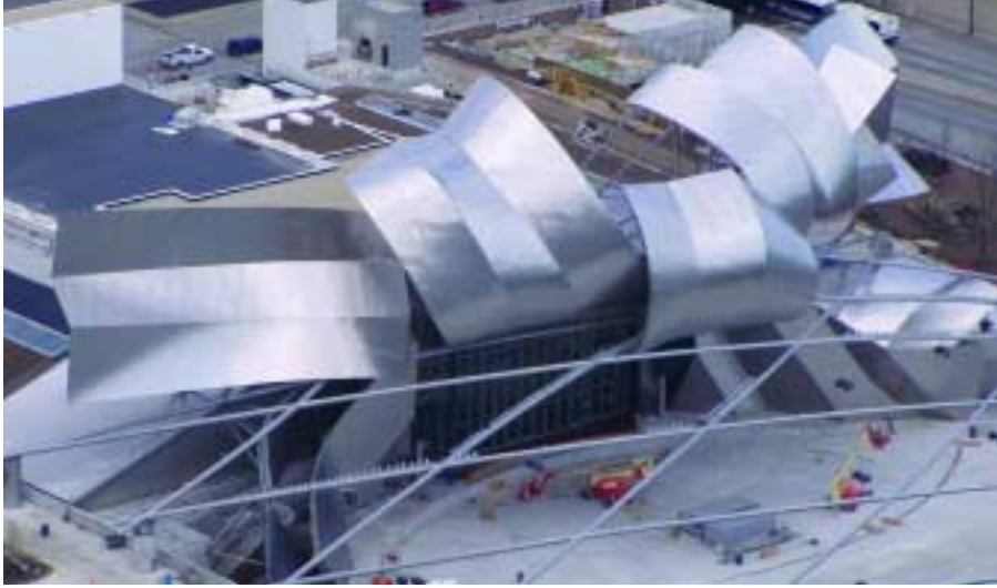
Curved stainless steel panels frame the stage opening at the Millennium Park band shell.
