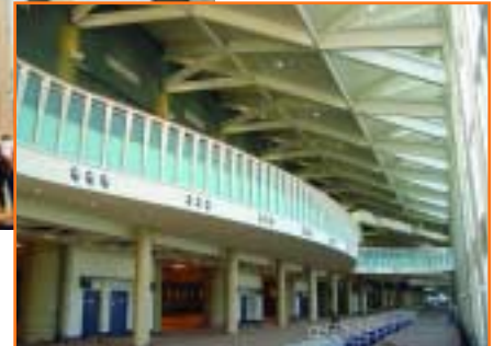
Above: The steel structure of the roof over North and South concourse takes a leading role in the finished architecture (inset, right).
