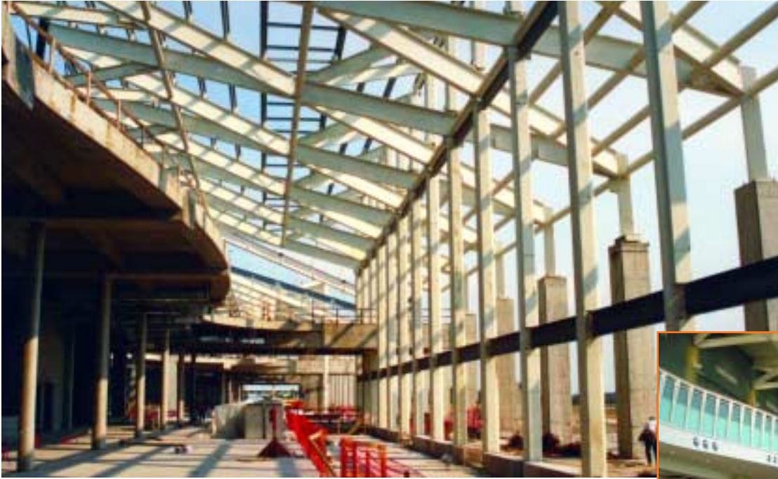
Above: The steel structure of the roof over North and South concourse takes a leading role in the finished architecture (inset, right).
