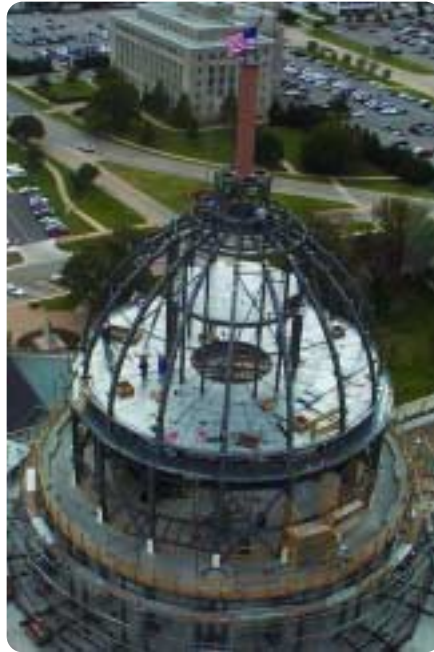
Photo courtesy Capitol Dome Builders.
