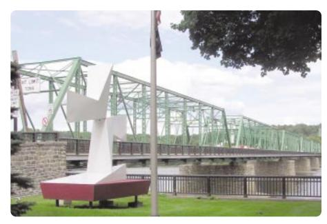
consists of six-span, pin-connected Pratt-type trusses, which are 27 ft high. Floor beams support roadway stringers with a 5"-deep open grid steel flooring. A cantilevered, well-used sidewalk resides outside the downstream truss.
