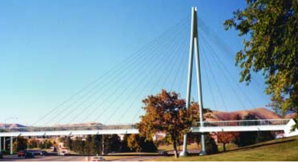
Dazzling steel cables splash a bit of flash into one of Salt Lake City's pedestrian bridges.
