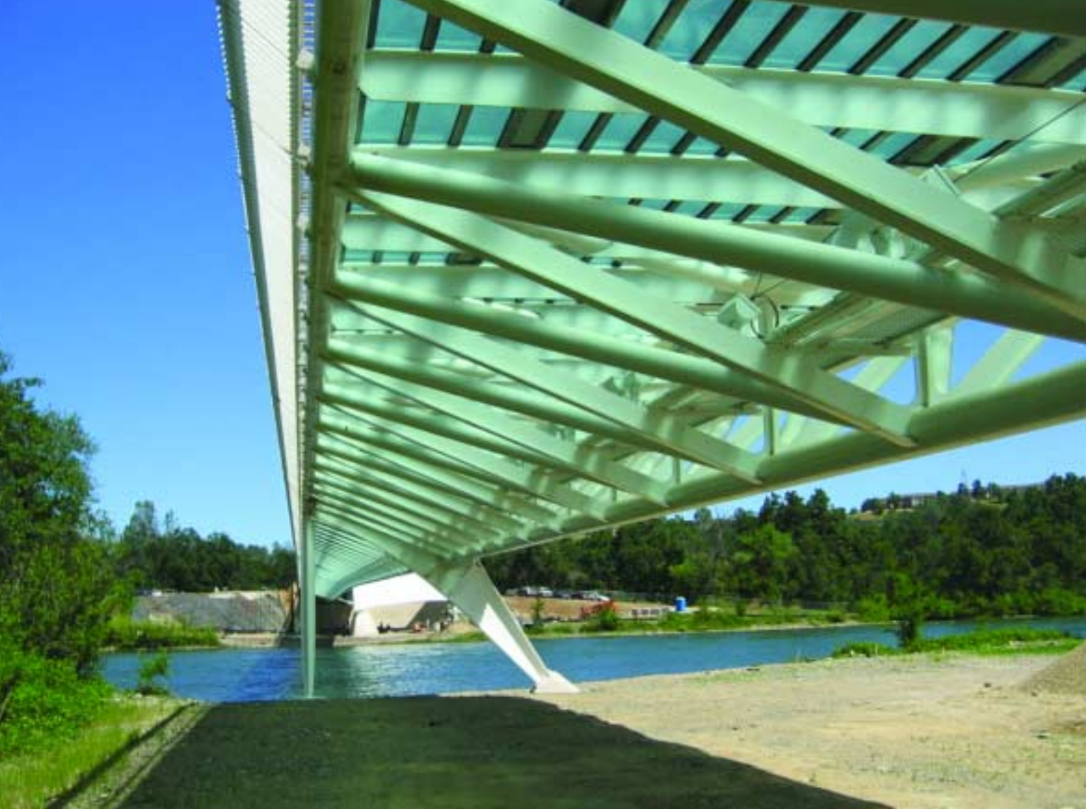
The bridge deck consists of translucent glass panels with granite accents.
