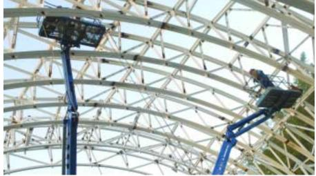
Above: Much of the structural steel is exposed on the underside of the shell. Note the many attachment points for performance-related rigging and equipment. (Photo courtesy Milco Constructors.)
