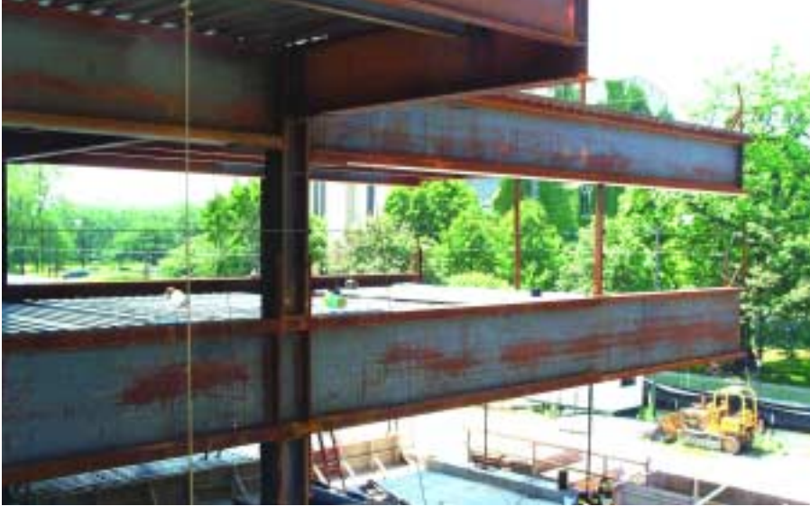
These plate girders for the dean's suite cantilever 42'.
