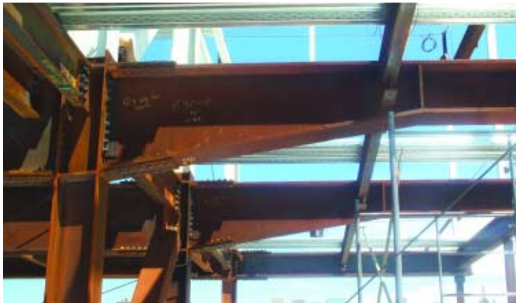
Below: Many of the cantilevers feature moment connected tapered plate girders.
