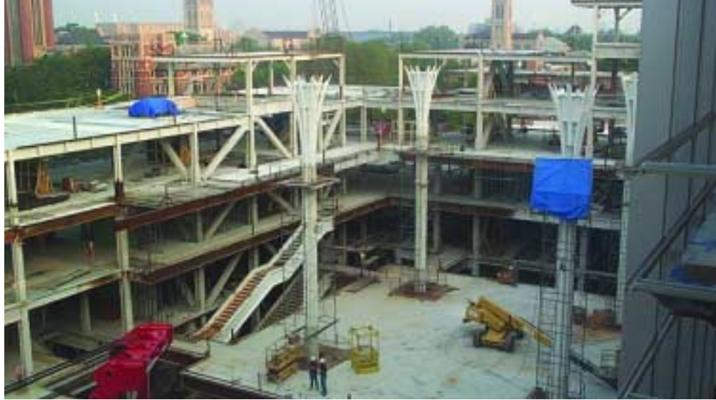
Above: The eight round sections of each main column branch out to become roof rafters in the Winter Garden.
