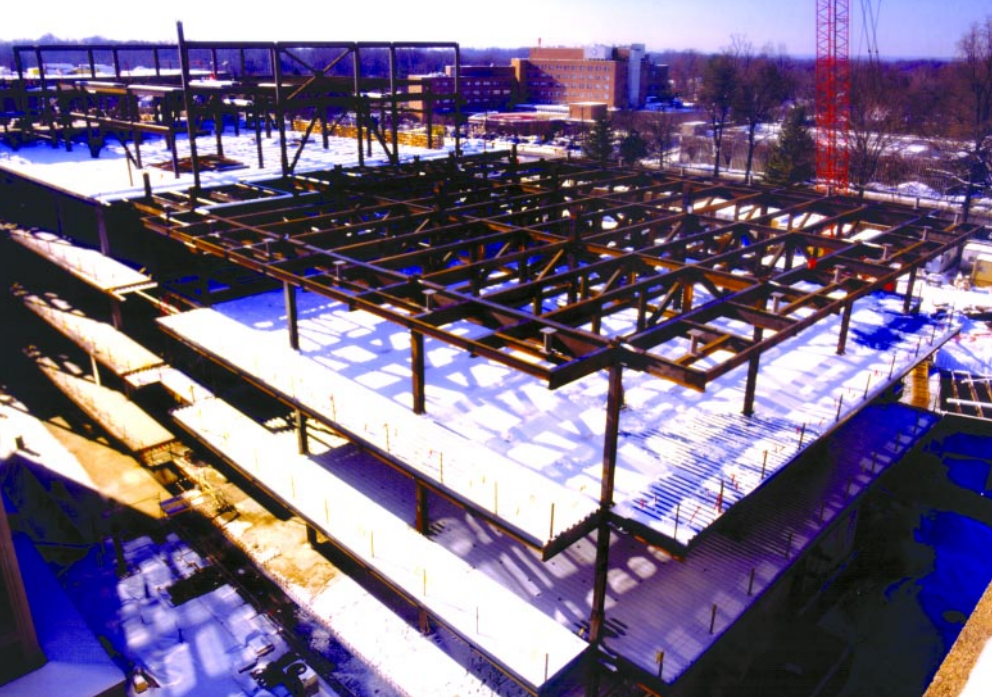
Phase 1 of construction of the Porter Center during erection of the trusses.
