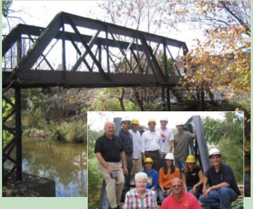
Top: VU's "Kissing Bridge" in its new location, prior to installation of the timber deck and guard rails.
