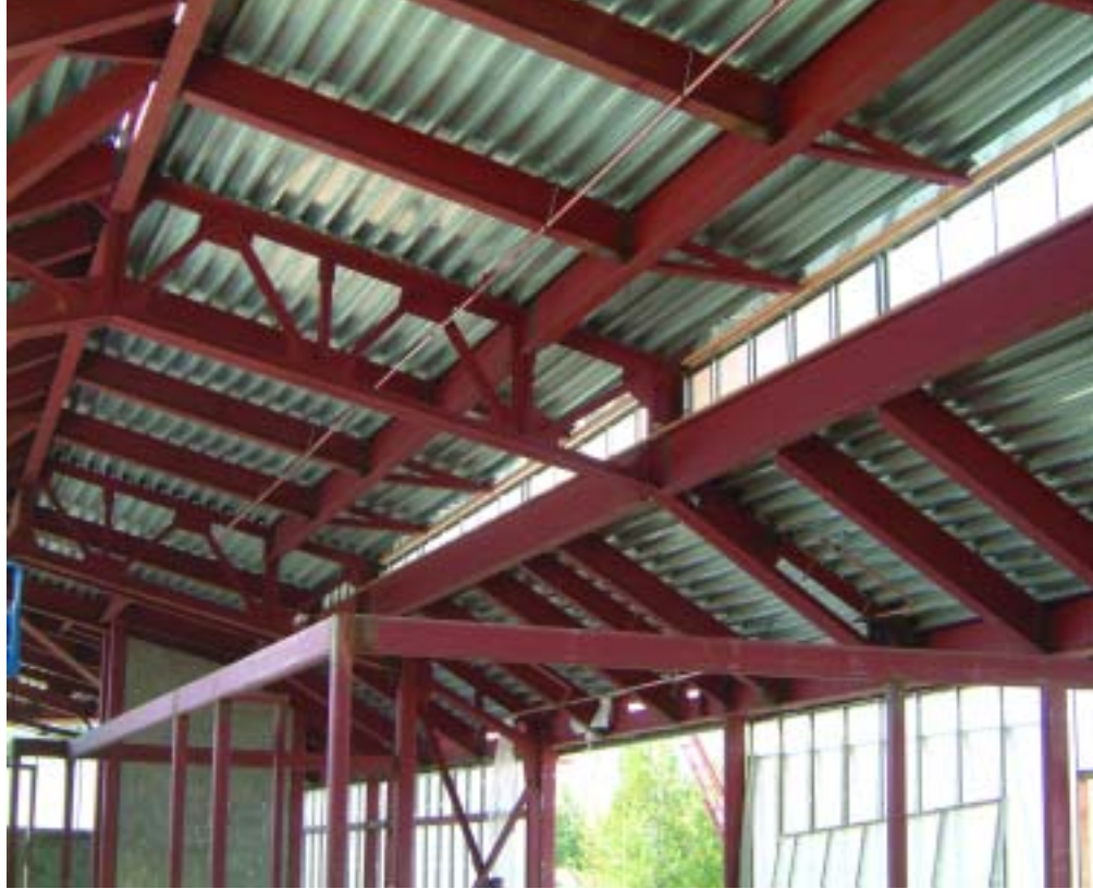
Above: Steel trusses (in the east-west direction) are the principal roof framing elements. They cantilever over columns on the west facade (at right in this photo) to provide a roof overhang.
