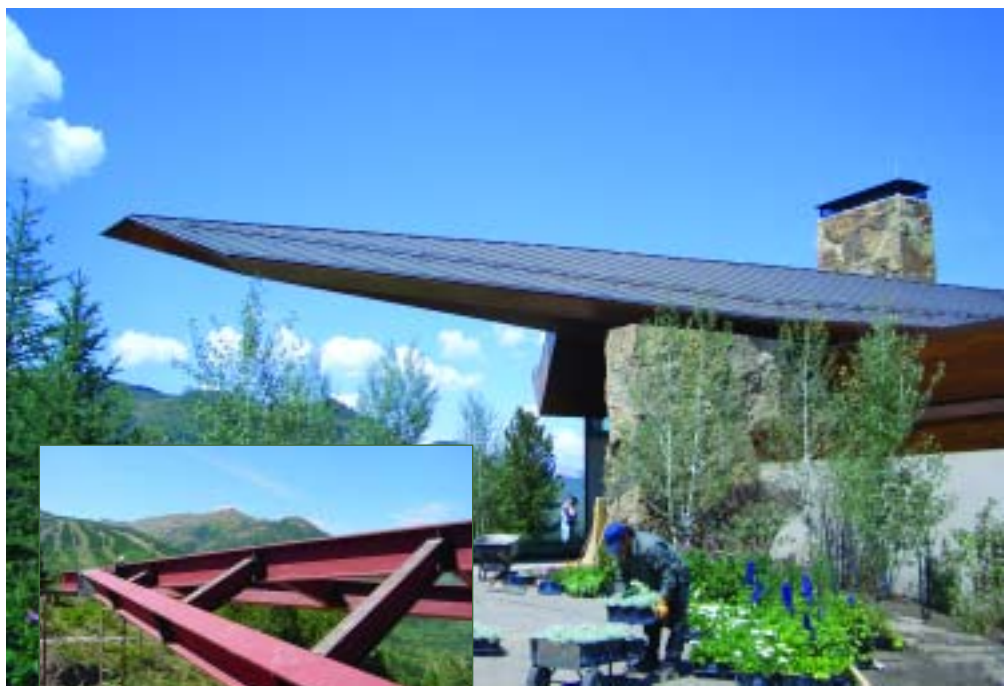
Below: The entrance canopy on the south end of the house is a 40' cantilever extension of the steel-framed folded-plate roof. The cantilever is framed with W shapes ( inset ).
