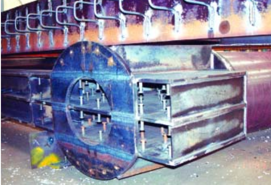
Transfer truss top-chord members were left open for concrete placement.
