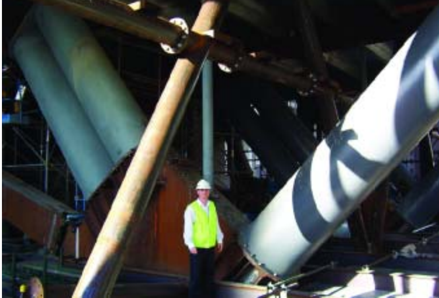
This photo provides a sense of scale for the two-story transfer trusses. Some of the two-tube diagonals used 1100 mm (43") tubes.
