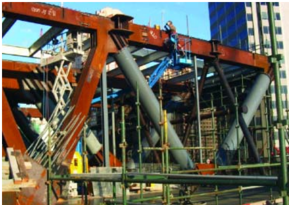
Two story transfer trusses transmit the tower column loads to the existing reinforced concrete structure below.
