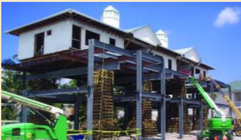
The first floor of the original cottages was demolished ( above ) before raising the remaining structure and inserting a new two-level steel frame underneath ( below ).
