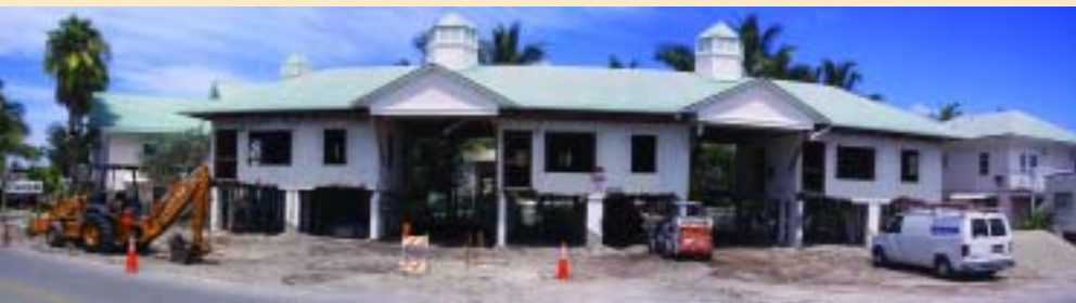
The first floor of the original cottages was demolished ( above ) before raising the remaining structure and inserting a new two-level steel frame underneath ( below ).
