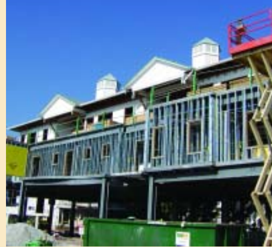
The second floor of the original cottages became the third floor after the renovation. All new infill construction used light gauge steel. "Hurricane clips" and straps were added to all existing wood framing.
