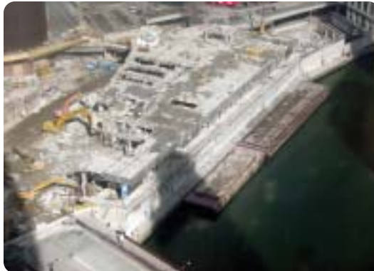
The old Chicago Sun-Times building (seen here in February, demolished nearly to street level) is being razed to make way for a 90+ story residential tower.
