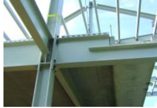
Steel framing supports precast concrete seating risers.
