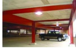
W-shape columns are smaller than most columns in concrete parking structures, contributing to the open feel of the structure while reducing door "dings" and enhancing safety.
