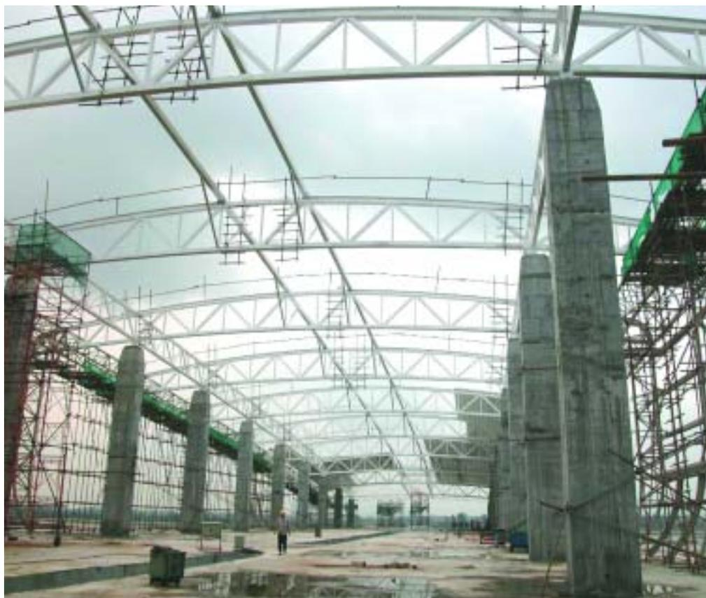
The central spine of the airside concourses consists of curved, planar HSS trusses spaced at 12 m (39'), supported by massive concrete columns.
