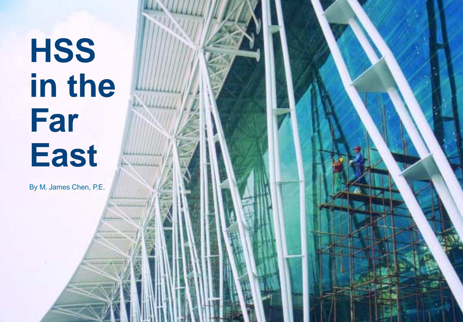
The main terminal features tilted and battered HSS columns of varying cross section, composed of three pipe shapes with plate stiffeners.
