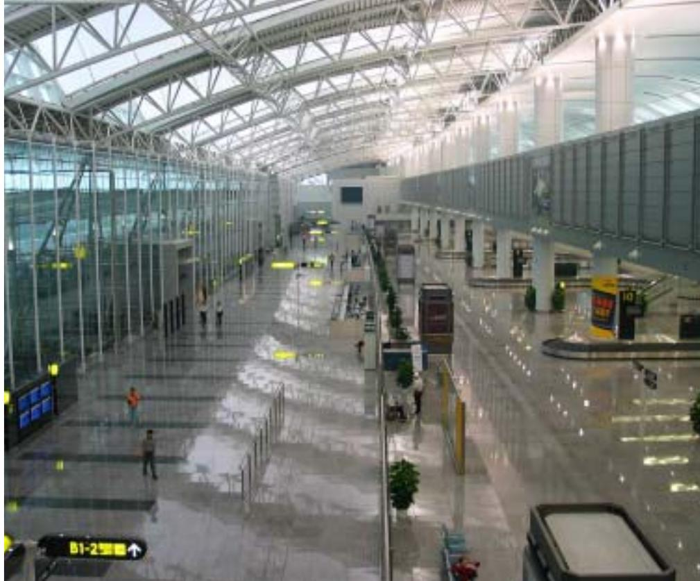
Triangulated trusses composed of round HSS create a dramatic interior space in the baggage claim area.
