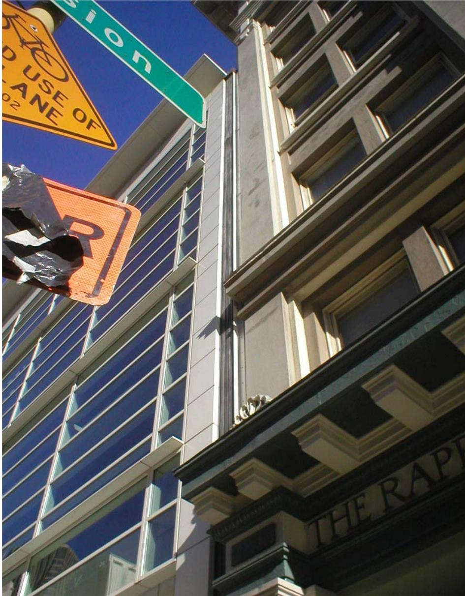
*Seismic Joint Between Adjacent Buildings*
