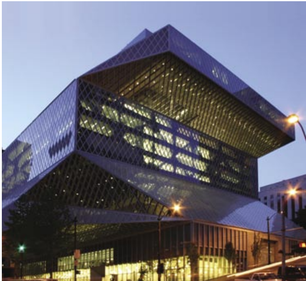
Photo by Michael Dickter, Magnusson Klemencic Associates.
