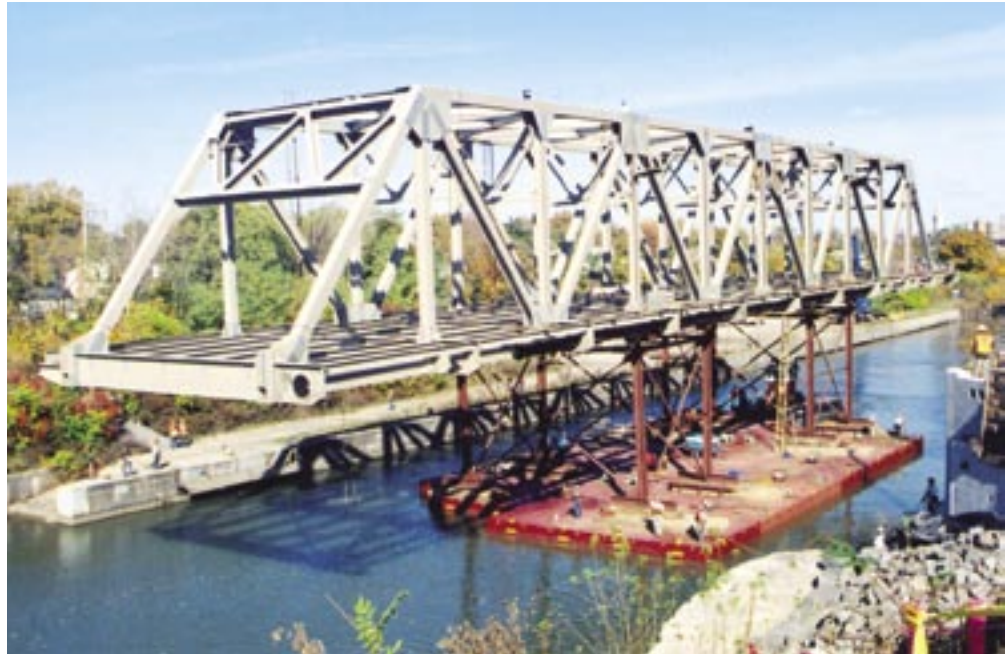
Floating the fully assembled bridge into place.
