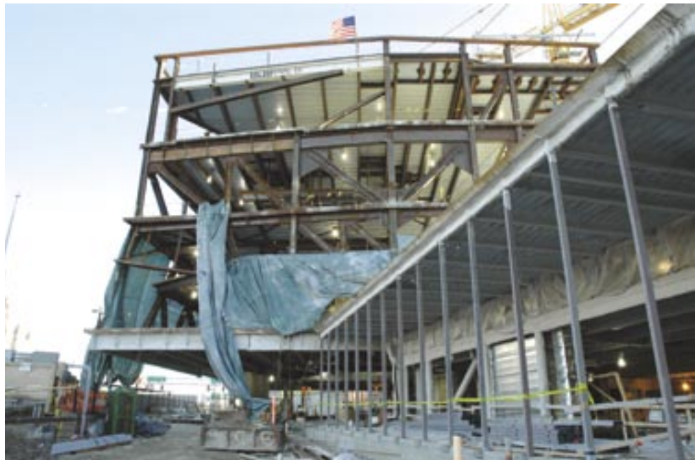
In this photo, the erection columns have been removed from the lower level, transferring the structural loads into the multi-story trusses.
