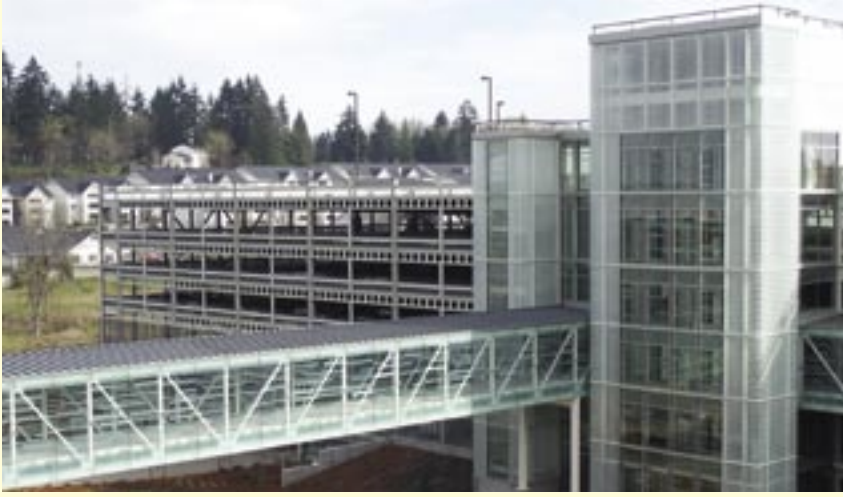
The parking structure features glass and steel exterior cladding that required tight tolerances for the steel frame.
