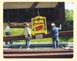
The Connector, certified to 57,000 lb, with a safe working load of 36,600 lb, has a fail-safe system in place—even if the hydraulic lines are cut, the load stays clamped securely in place.
