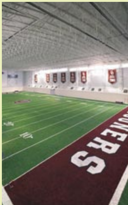
Steel deck and joists by Nucor Vulcraft Group.
