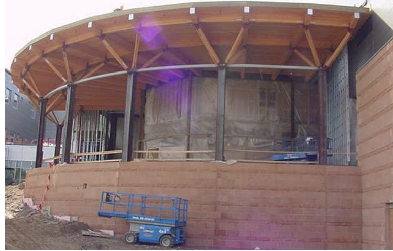
This page: The extensive use of wood framing for the Community Center's roof required that it be structurally isolated from the rest of the hospital to meet fire code requirements. Photos courtesy Hammel, Green and Abrahamson, Inc.
