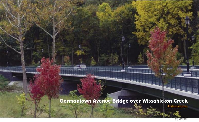
he Germantown Avenue Bridge over Wissahickon Creek in Philadelphia is a three span curved steel girder bridge that was designed to safely replace a failing nine span straight bridge.
