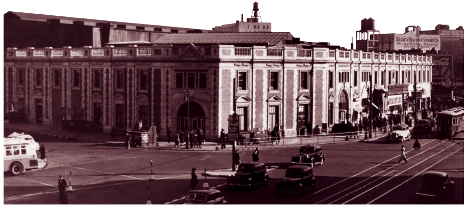
The original Flatbush Avenue station, constructed in the 1920s, was demolished in the 1980s, but original structure remained in place below street level.
